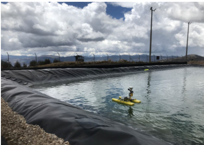
Conducting a Bathymetric Survey to Verify the Volume of a Process Water Pond
