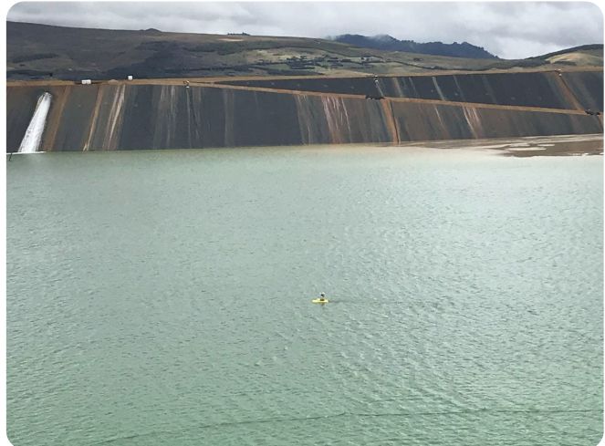
Figure 6 - HyDrone-ASV Surveying the tailings pond.
